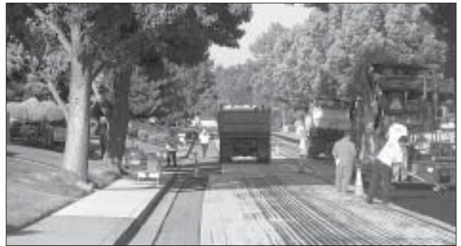
Street maintenance was a high priority in 2005 and 2006. Here, Encina Camino gets an overlay. Carleton Thompson
