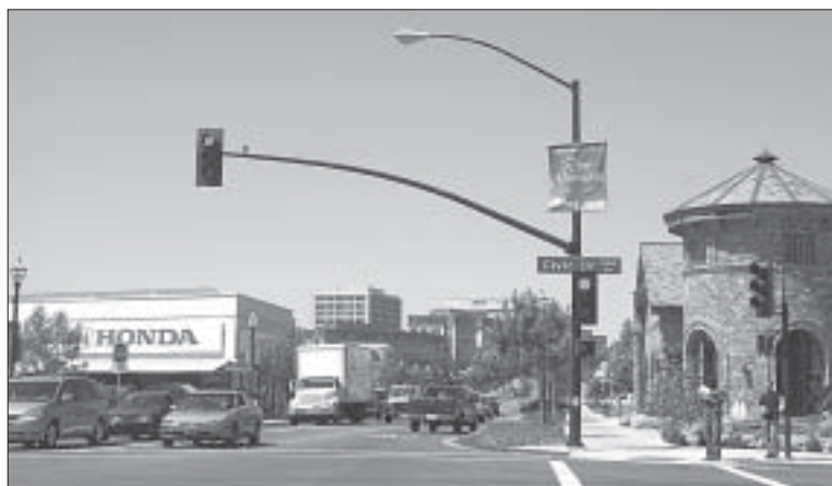
MAIN STREET'S FACELIFT COMPLETED — Following 10 months of construction, the City in February 2005 finished the makeover of North Main Street between Civic Drive and Ygnacio Valley Road. The $2.4 million cost will be shared by adjacent property owners on Main Street. The finished project involved the removal of power lines and utility poles and the addition of attractive new landscaping, walkways, lighting, and pedestrian-friendly crosswalks.
